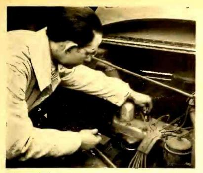
Quiet reception is assured at all times when suppressors are used at the spark plugs. Continental Carbon's new 5000-ohm low-resistance units don't reduce engine efficiency.
