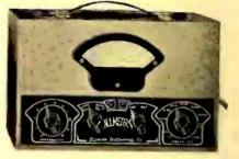
★ AC-DC operated instrument measuring AC and DC volts 0/15/150/750. On AC non-reactive to 10 megacycles. Capacity ranges .001 to .1, .1-32 mfd. Resistance—.03 to 500, 500 to 5 megs. Inductance 2-1000 henries. Housed in wrinkle-finish shield cabinet. Weight 4 pounds. Superior Instruments Corp., 136 Liberty St., New York, N. Y.— RADIO TODAY—see aso advt. p. 69.
